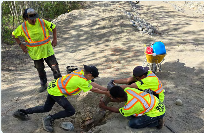
Trail construction and maintenance
